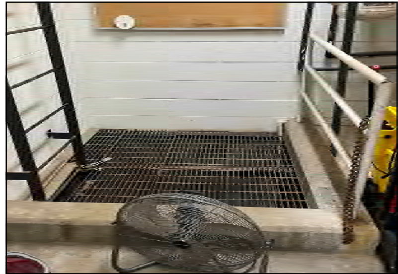
6) View of inaccessible pump house located in the maintenance area.
