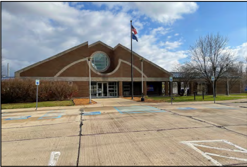
1) View of Clear Creek Welcome Center main building.
